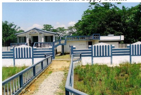
Salchakra Part-II Water Supply Scheme
