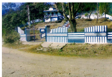
Kalaincherra Water Supply Scheme
