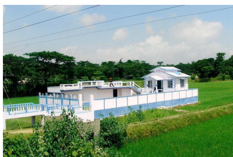
Srikona Part-II Water Supply Scheme
