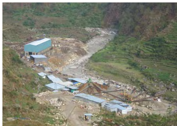
Bhilangana-III : Stone crusher
