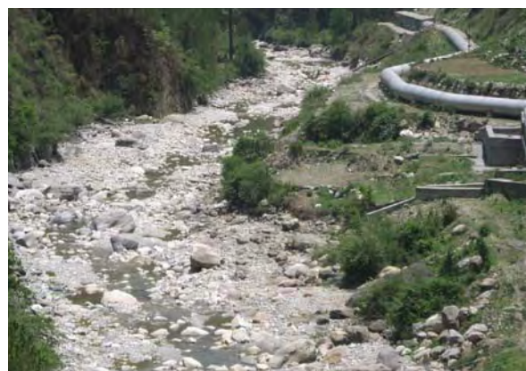
Debal - Downstream flow; Penstock is seen parallel
