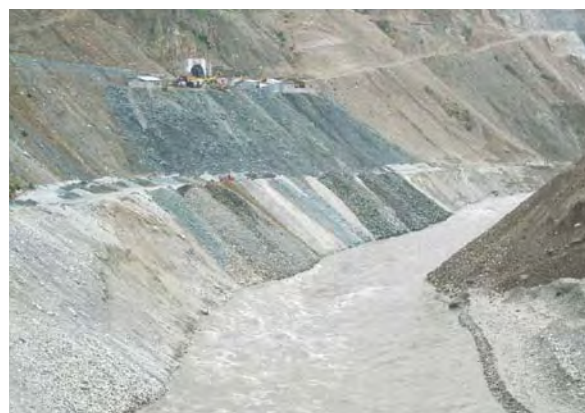
Srinagar project on river Alaknanda - Muck disposal
