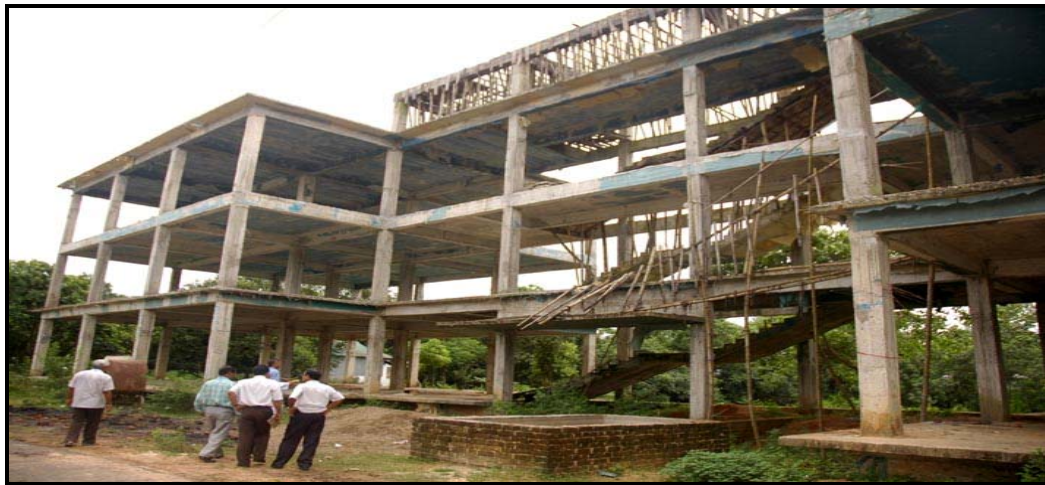
View of the incomplete building of Bhavan's Tripura College
