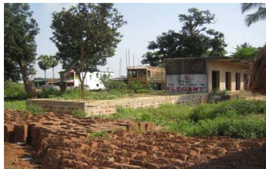
Market Complex at Nagapur Bazar(GOP PS)
