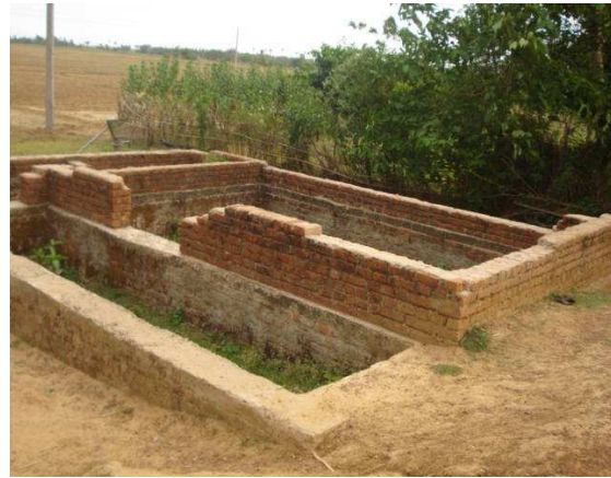
AWC building at Sasanpada, GP-Chikana (PS Binjharpur)
