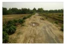
roads constructed at a cost of Rs 13.86 crore were non-durable and below the Grade I metalling level. Joint physical inspection in the
