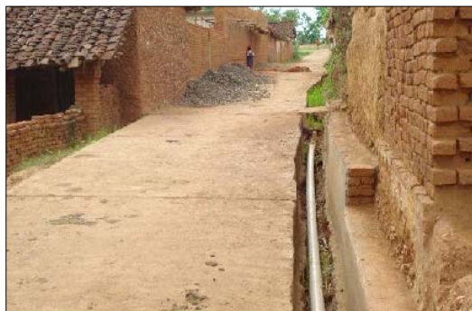
View of pipeline laid in existing drain of cement concrete road in village Khamha for which cutting of cement concrete road was shown. (Spot: main road Khamha village, August 2009)
