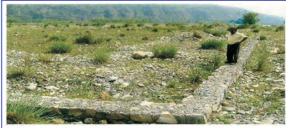
Abandoned work of Solid Waste Management Project after incurring expenditure of Rs 0.83 lakh
