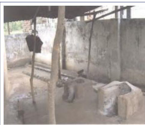
Kitchen for Mid-Day-meal in the open in a temporary structure in GMS, Bohlion
