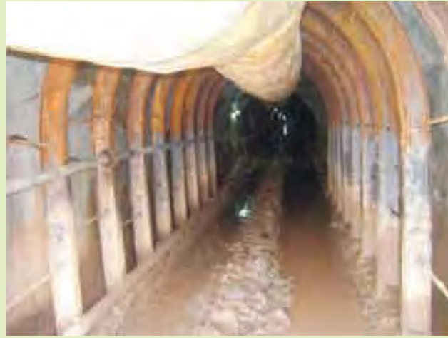
Tunnel work (inner side) in progress in Medium Irrigation Project, Sidhata
