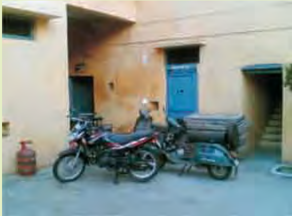
Traffic, Tourist and Railway PS at Amb without basic amenities like parking, reception room, etc.
