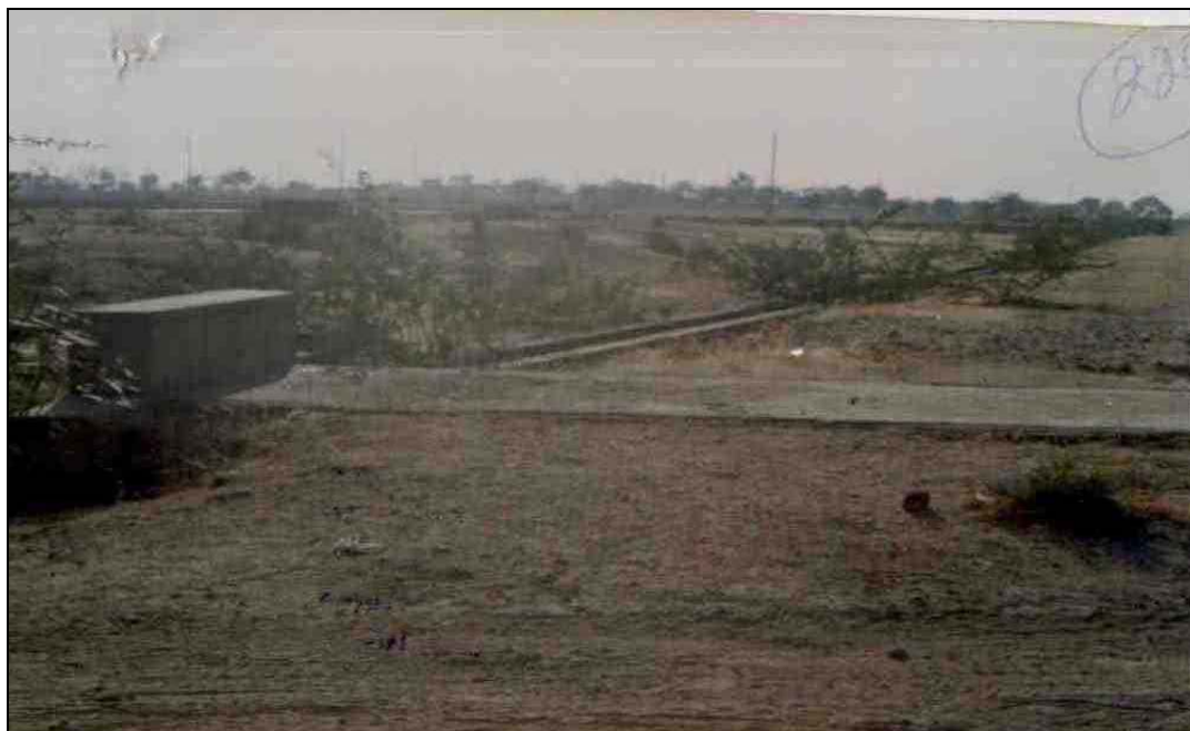
Views of incomplete project works at Bandanwara village
