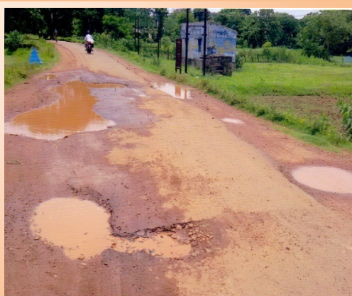
Potholes developed on Marthapur-Jamunakote road due to non-maintenance of road Dhenkanal district, Odisha
