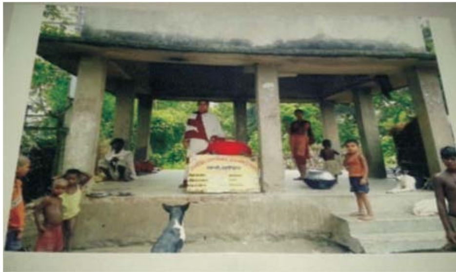
Anganwadi centre (no. 146 of Barari, Katihar) running without basic infrastructure.
