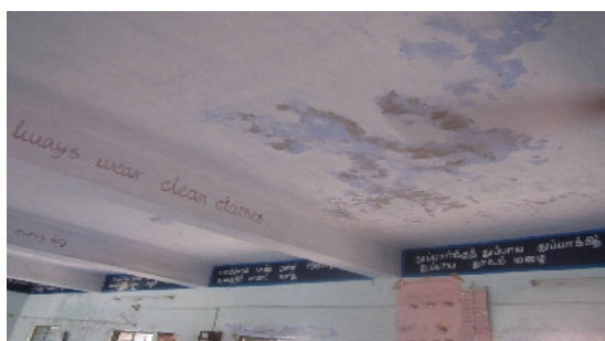
Picture 2: Poor condition of ceiling in a classroom in S.Kovilpatti PU Middle School in Singampunari PU
