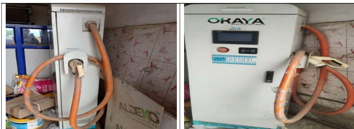
Picture 3: Shiv Filling Station, Solan, Himachal Pradesh Chargers removed from installation site
