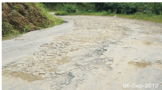
Stone filling and Water logging in Pot Holes in Lunglei – Tlabung Road (9.00 - 39.00 kmp)
