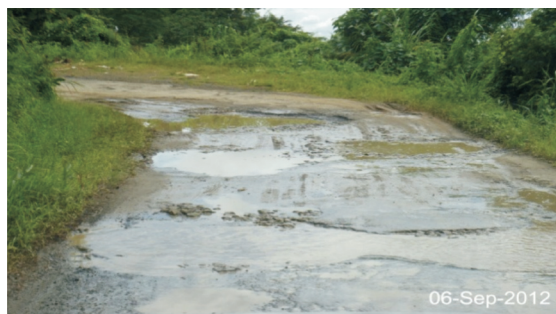
Stone filling and Water logging in Pot Holes in Lunglei – Tlabung Road (9.00 - 39.00 kmp)
