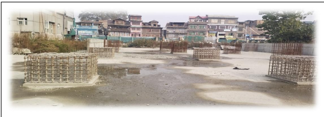
Incomplete works of extension Block of Lalla Ded Hospital, Srinagar
