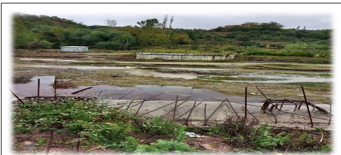
(Bridge at Waz Mohalla, Kreeri over Frestahar Nallah to which approach roads were yet to be constructed)
