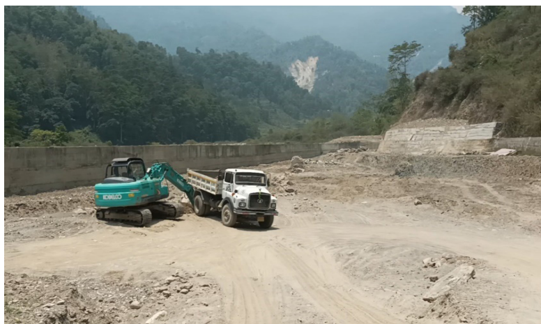
Image 7.26: Sipchu landfill Under Construction
