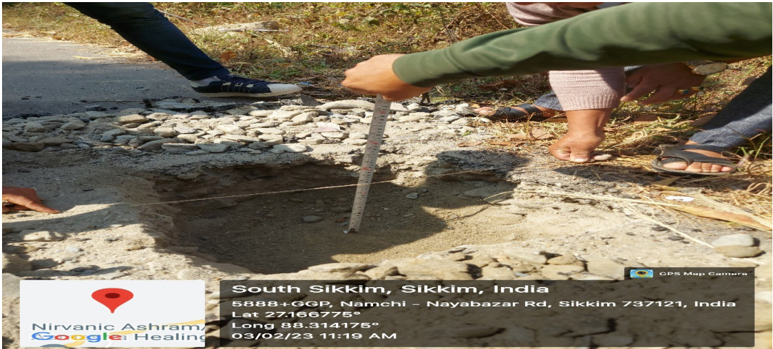
Thickness test at Dong Ambotey School to Approach road to Adhikari gaon
