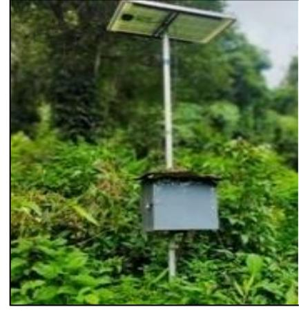
**Figure 2.6:** Non-functioning solar fence - Bimaram in Ranni range (23 September 2021)
