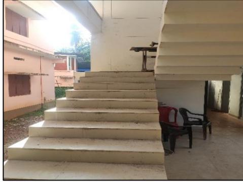
**Figure 2.13:** GHSS Parayanchery, Kozhikode - stair without handrails provided
