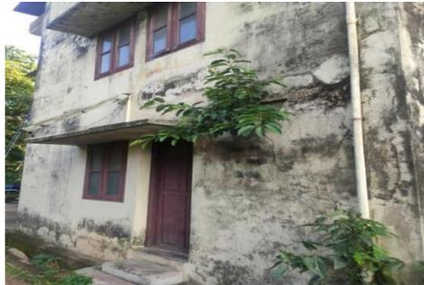
**Figure 2.19:** Cracks and vegetation growth in Pavamani Quarters, Kozhikode
