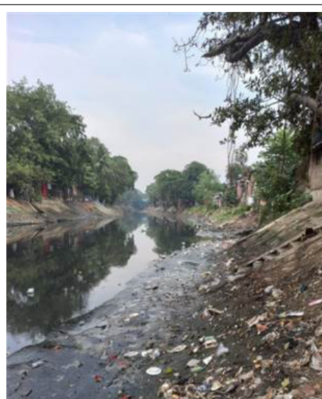
Figure 4.13: Dredging work yet to be started
