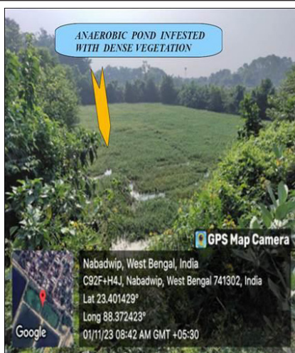
Figure 4.7: Anaerobic Pond infested with dense vegetation
