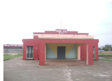
Renovation of Town Hall, Subarnapur
