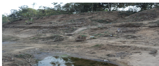
Embankment in Subarnarekha River not restored
