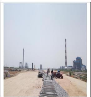
Picture No. 2.1.2:Track laying in RSMY works
