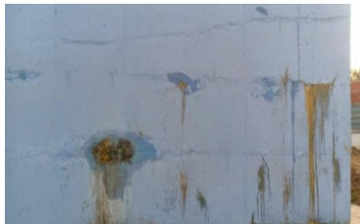
*Damp and crack at Beur STP*
