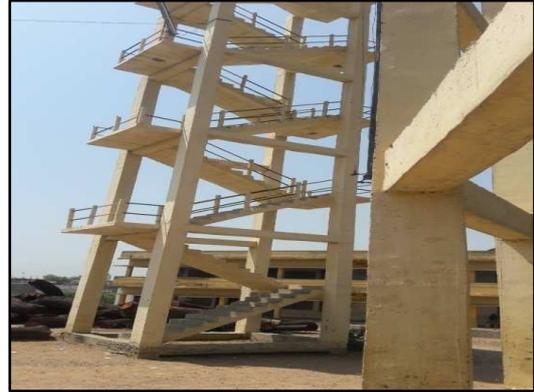
*Non-provision of railings to stair case of 1<sup>st</sup> and 2<sup>nd</sup> flights of ELSR*
