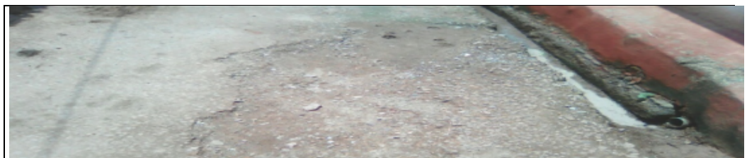
Connectivity road along with drains from school to Mangilal Jat house Gobercha (GP, Sakrawada)
